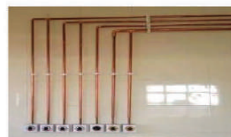
Medical Gas Pipeline System
